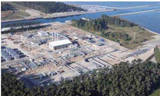
The shore station of the Nord Stream pipeline in Lubmin near Greifswald
